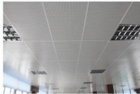
SoundTex吸音无纺布材料可直接贴在天花板上 SoundTex sound-absorbing nonwovens can be mounted without difficulty into ceiling systems.
