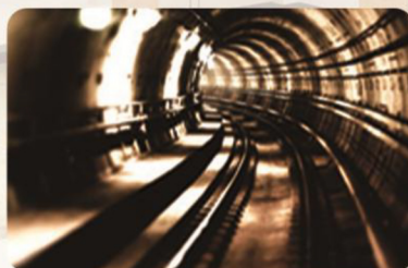
Yangtze River Tunnel Wuhan
