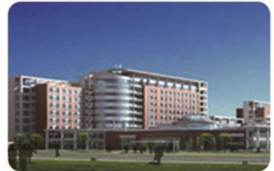
1st People's Hospital Chengdu
