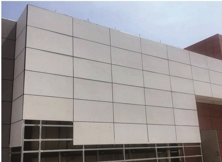
exterior wall works
