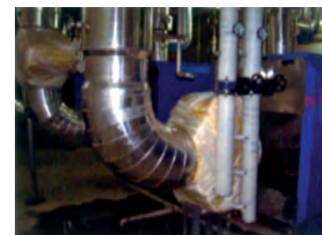
气体板式热交换器 Gas/liquid,plate heat exchanger
