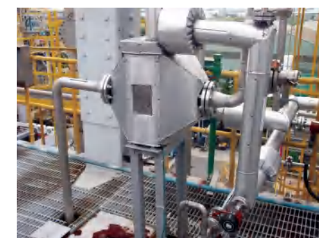
气体板式热交换器 Gas/liquid,plate heat exchanger
