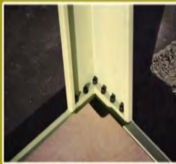
立柱与底梁连接 The Corner post jointed with the bottom beam
