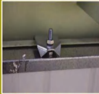
墙板的固定 Install method of wall panel
