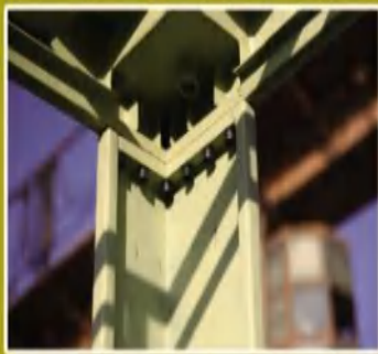
立柱与顶梁连接 The Corner post jointed with the top beam
