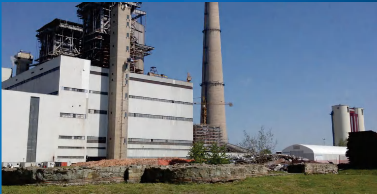
Power plant in Kostolac Serbia
