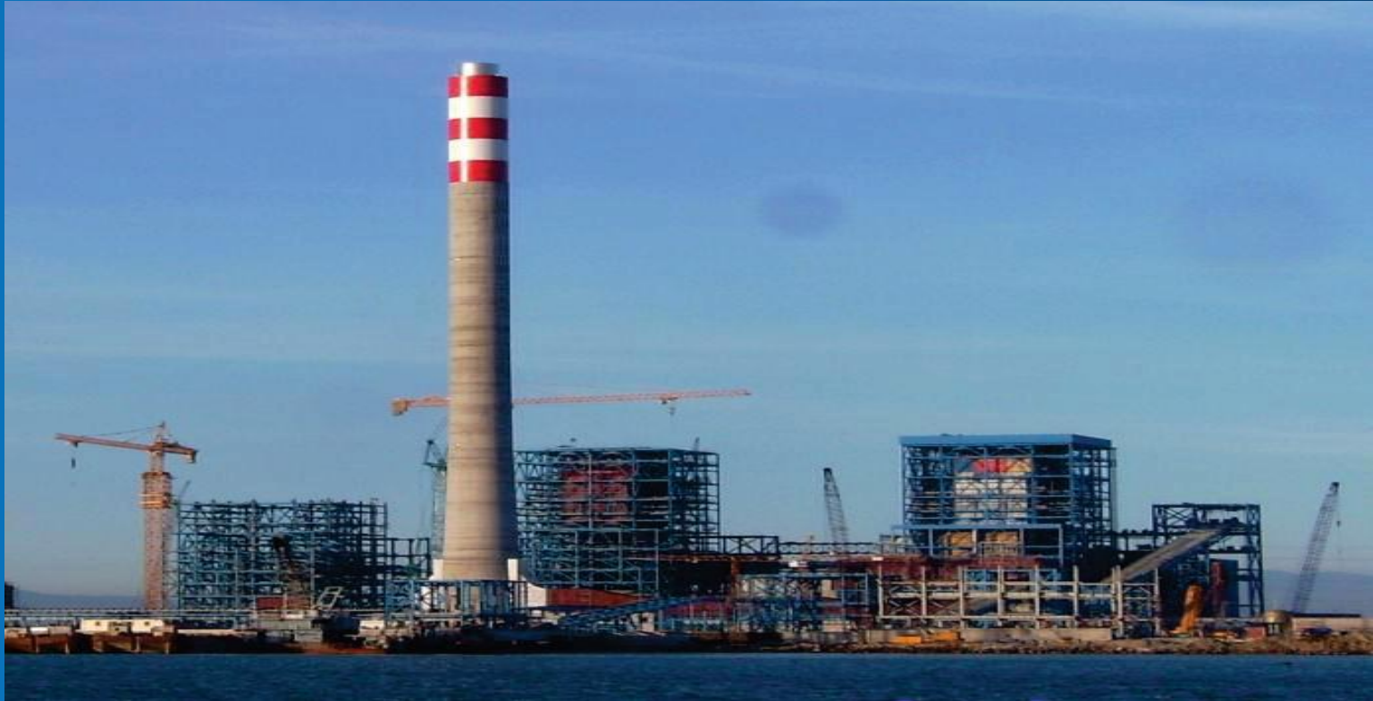
The steel structure project of 3*330WM power plant in Indonesia
