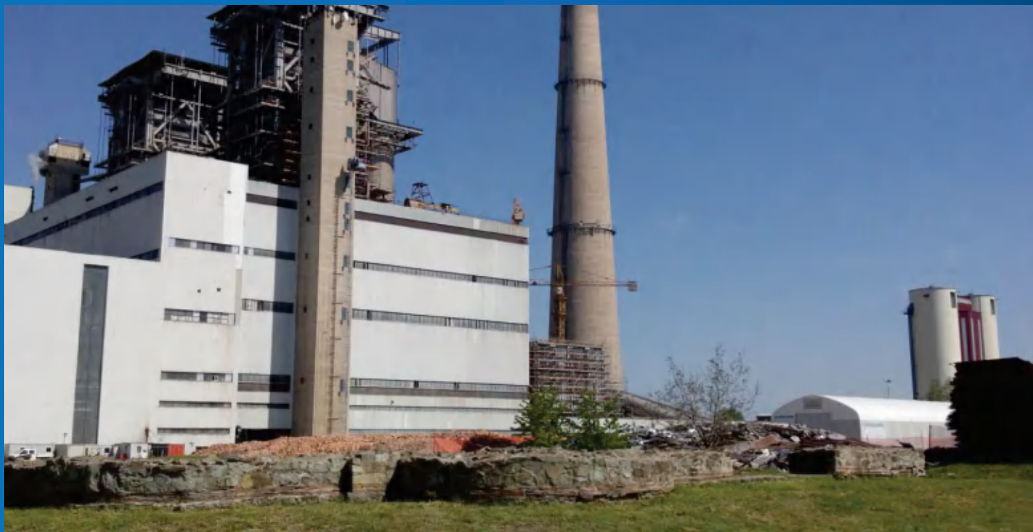
Power plant in Kostolac Serbia
