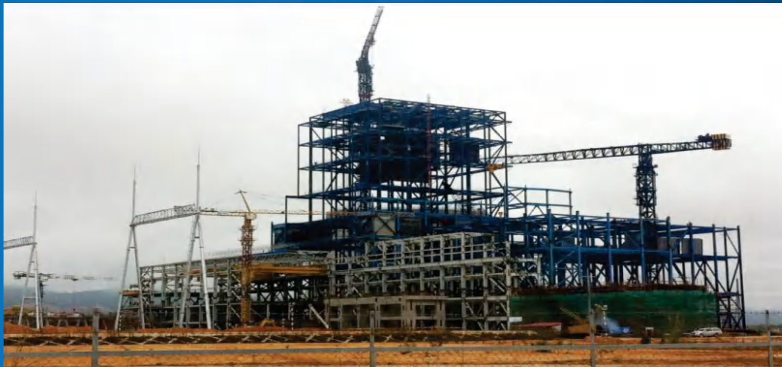
Laos hongsa power plant project
